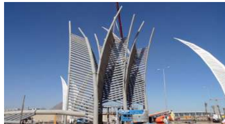
Fire Proofing and Painting
