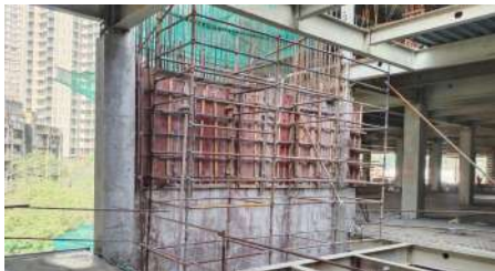
Civil & RCC Work
