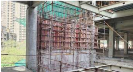
Civil & RCC Work
