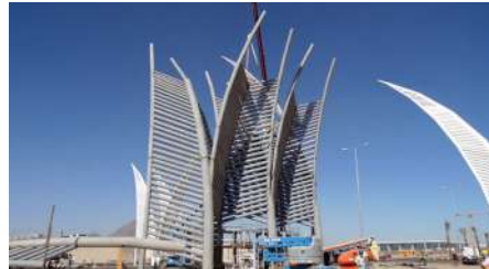
Fire Proofing and Painting
